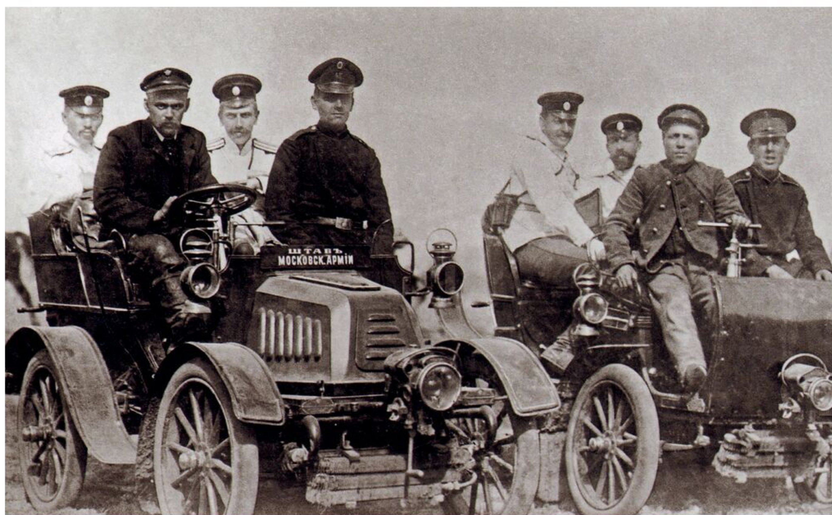
An 8-hp front-engined Frese and a 6-hp rear-engined Frese at Kursk.
